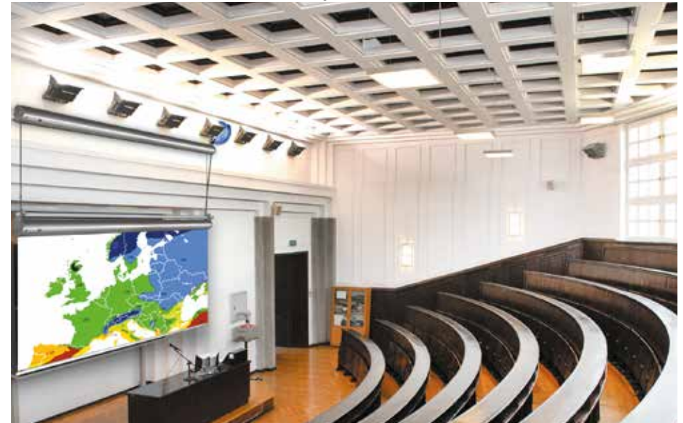
Lifts are able to lower projection screens to the level where they can be used even in
